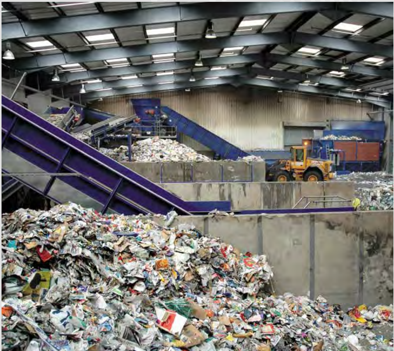
Reppie waste-to-energy plant, Addis Ababa, Ethiopia
