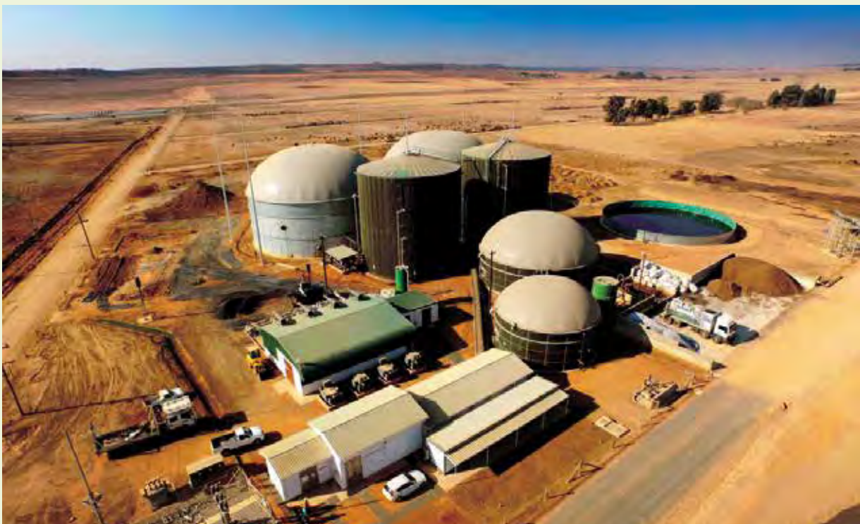
Bio2Watt biogas plant, Bronkhorstpruit
