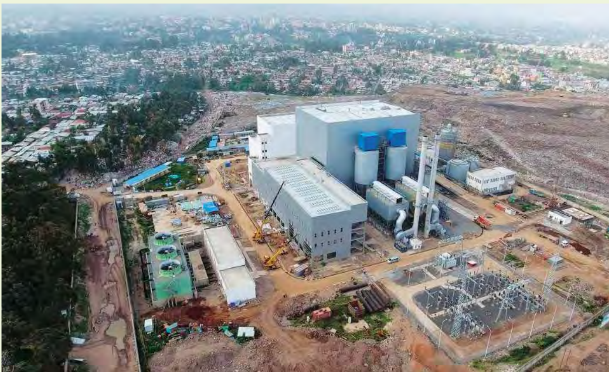
Reppie 50MW waste-to-energy plant at the Koshe dump in Addis Ababa, Ethiopia
